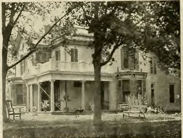
RESIDENCE OF HON. W. M. FOGLER. Corner Third and Randolph Sts.
